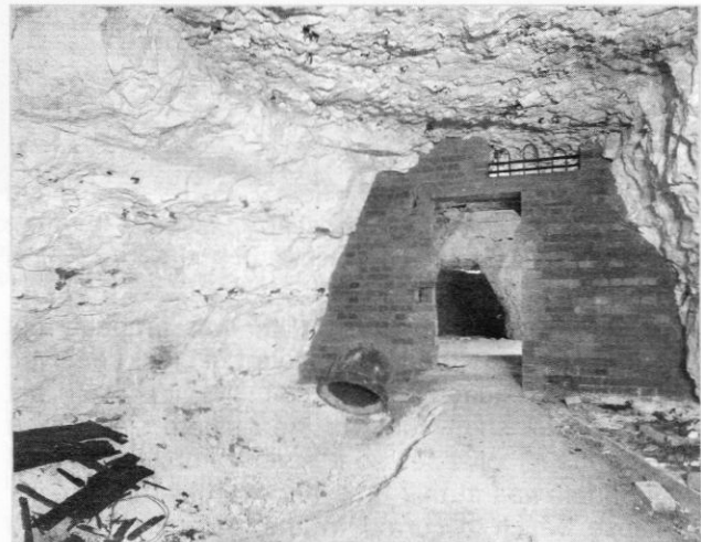
This picture shows the entrance to the council chamber from the inside. The large earthenware pipe to the left of the door is assumed to be part of the ventilation system. The humidity is always very high in the chalk mines and any material such as wood or paper will soon rot away.
